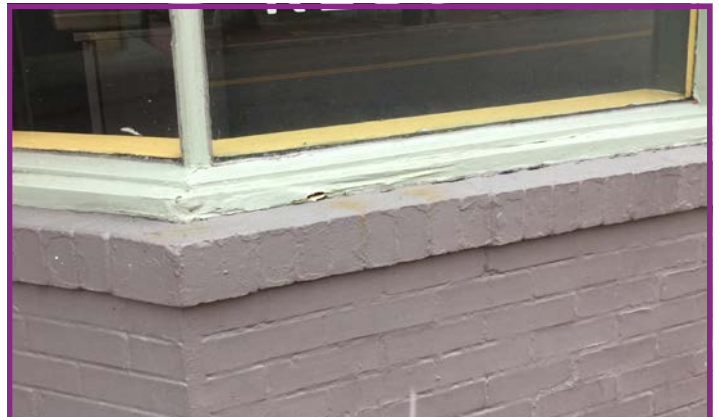
Inspect and Repair Wood Windows
