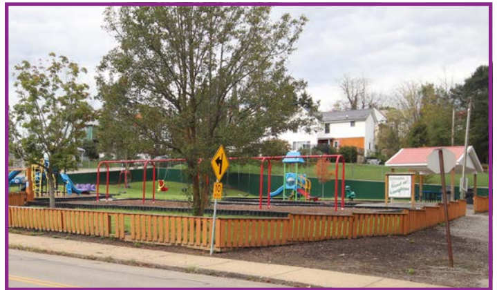
Harriott Avenue Playground's Playground Equipment and Fencing
