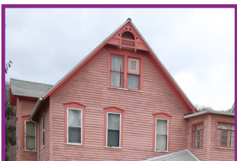
Steep, Front- Facing Gable Roof
