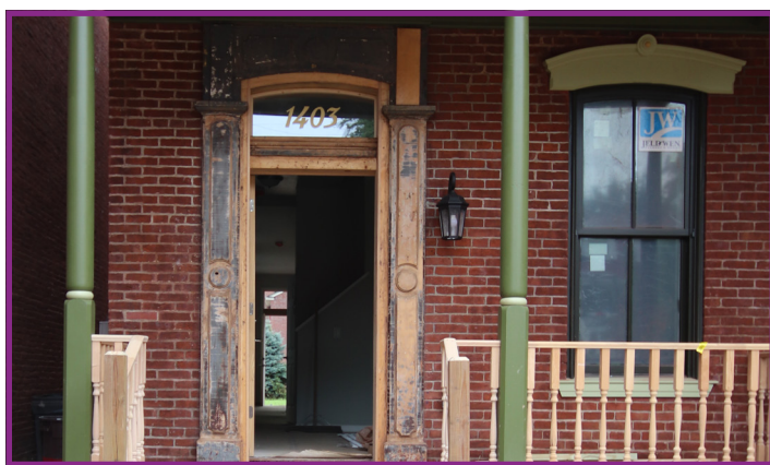
Preparing Wood Surface for Paint by Scraping and Sanding Wood
