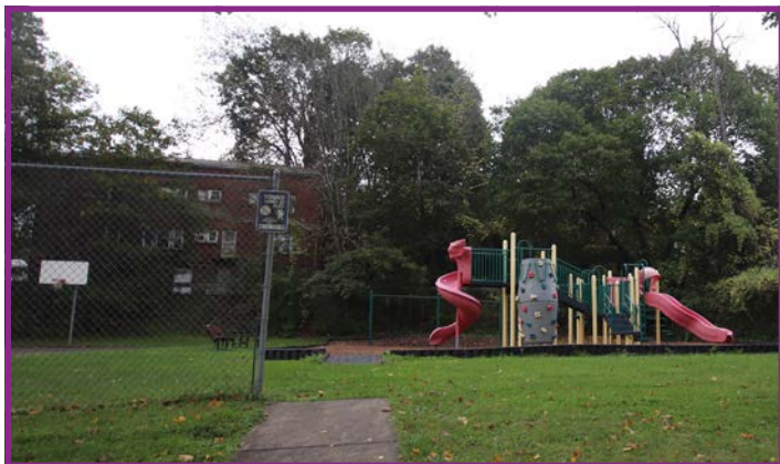
Innis Street Playground Basketball Court and Playground Equipment
