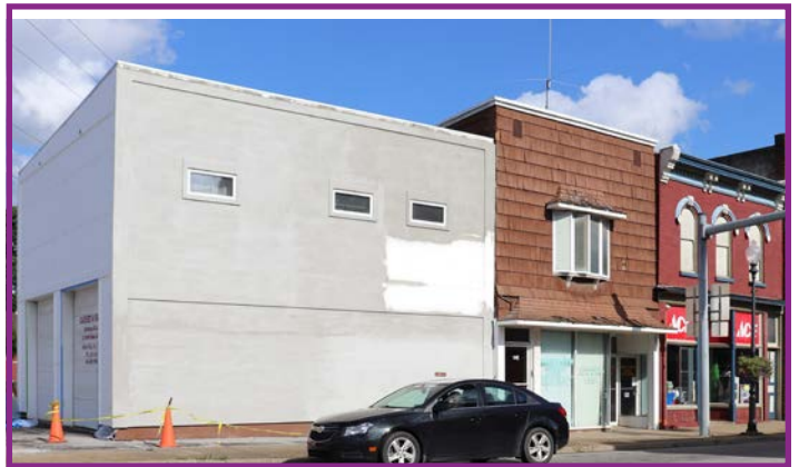
Inappropriate Frontage for Historic District, Entrance Removed on Main Street and Garage Doors on Side Street
