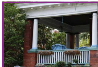
Masonry Pier and Column Porch
