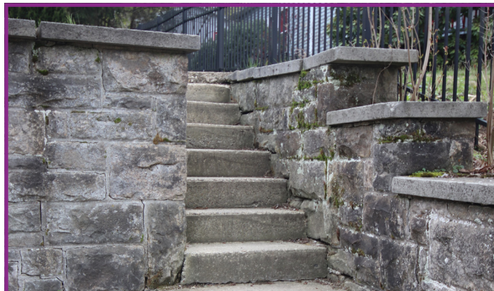
Steps Built Into Stone Retain Wall
