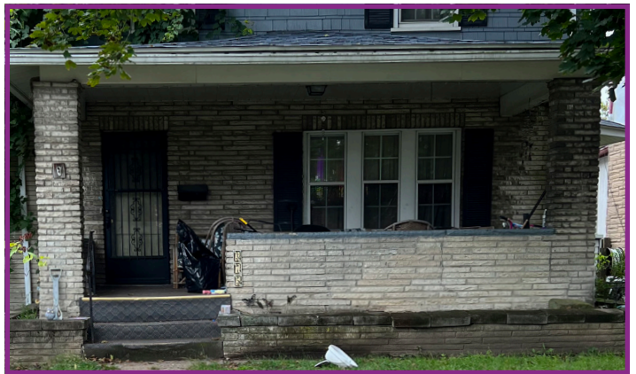
Dwelling Clad in Brick Veneer
