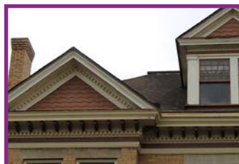
Cornice with Brackets and Dentils
