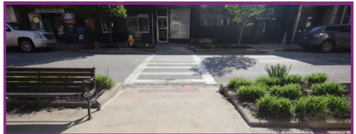
Accessible Crosswalk with Landscaping
