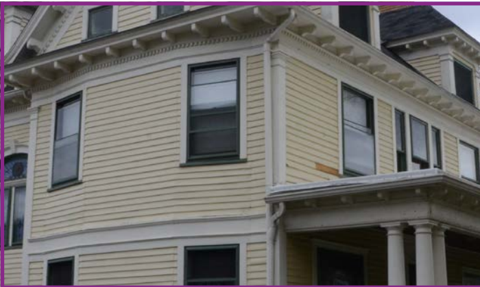
Wood Cladding and Rafter Tails
