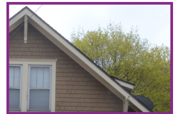
Wood Shingle Cladding
