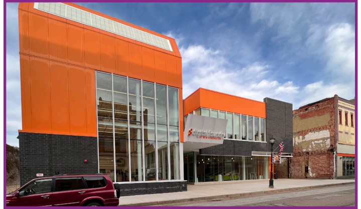
New Construction with Appropriate Building Massing and Height for a Historic District. Fenestration Patterns, Form, Setbacks, and Materials are Inappropriate
