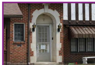
Round Arch Entry with Decorative Stonework
