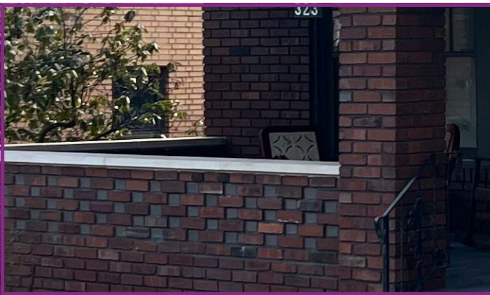
Rebuilt Railing and Column
