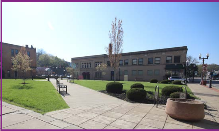
Town Square Looking Southeast
