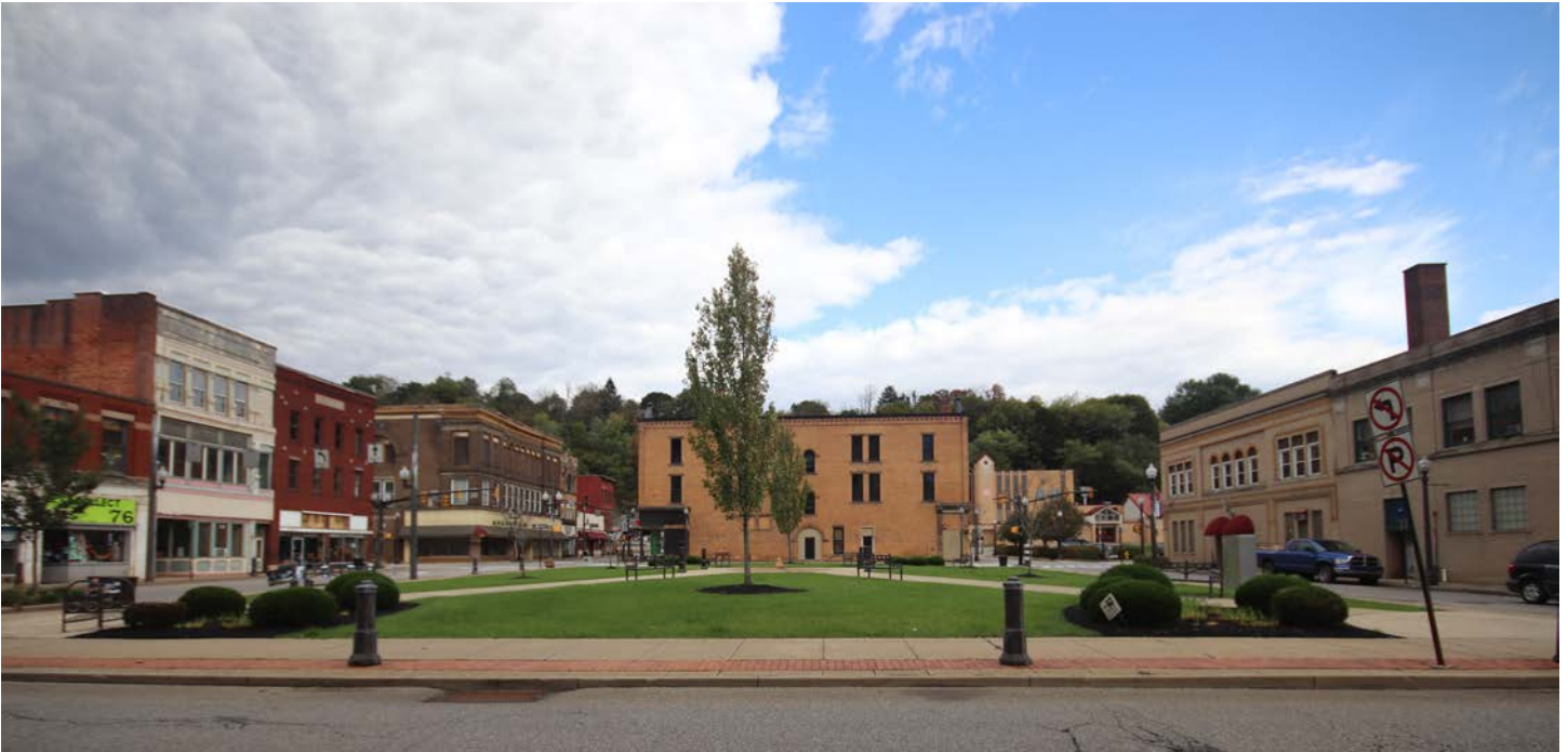
The historic Brody Block was demolished to make Oil City's Town Square, which is a public park and gathering space for community events.
