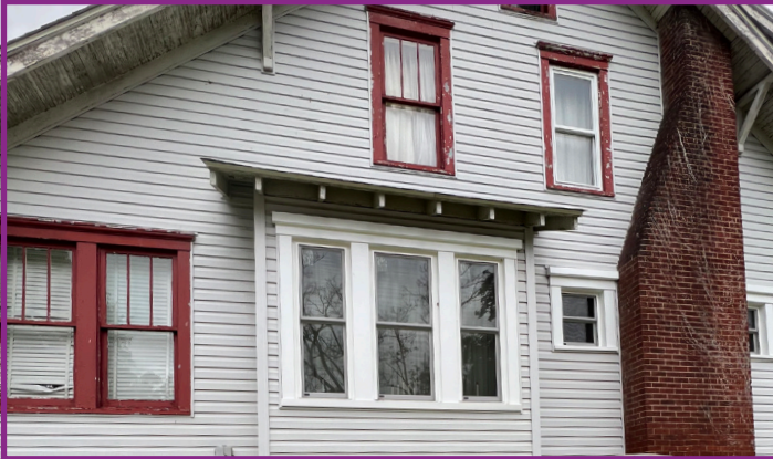
Inappropriate Window Replacement. Match Window Style with Original Style if Replacing or Restore Original Windows
