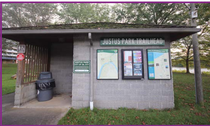
Justus Park's Existing Restrooms and Trailhead Information
