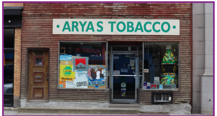
INAPPROPRIATE Fenestration Pattern and Window Style
