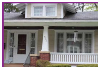
Exposed Rafters and Sturdy Columns
