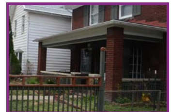
Massive Porch Columns
