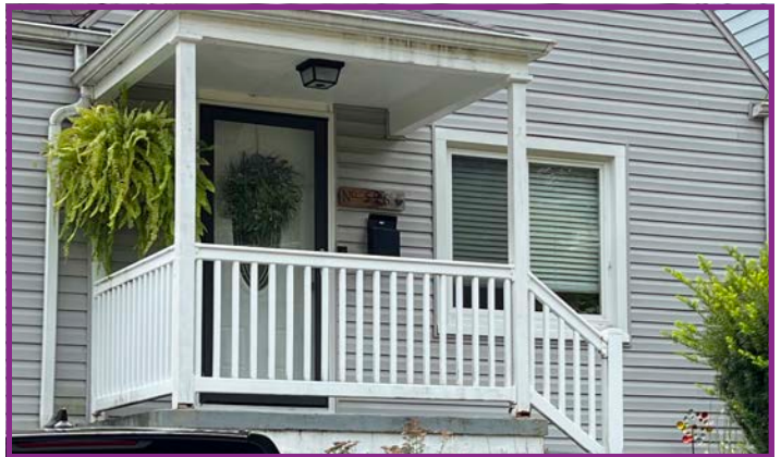
Vinyl Replacement Porch Columns and Railings Often have Incorrect Proportions and Styles
