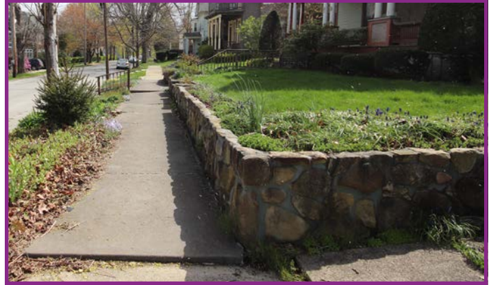
Stone Retaining Wall
