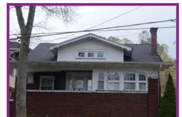
Low Slope Roof
