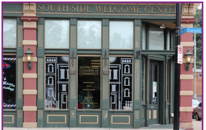
Transom Window on a Historic Storefront
