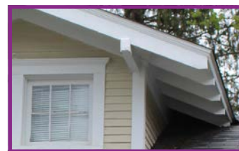
Exposed Rafter Tails
