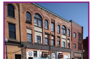
Masonry Construction with Stonework
