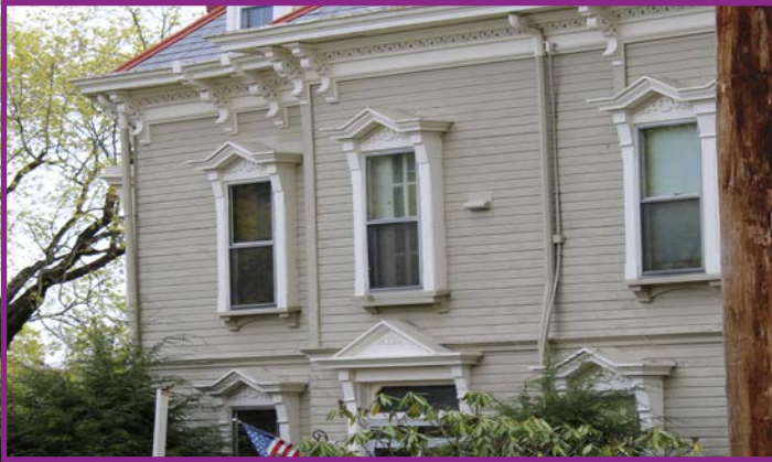
Original Wood Window Crowns, Brackets, Cladding, and Cornice
