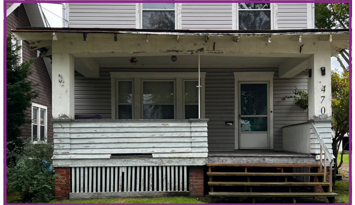
Wooden Porch and Cladding in Need of Repair
