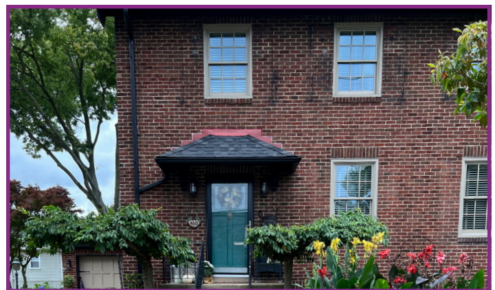
Gently Clean Masonry of Soot and Dirt
