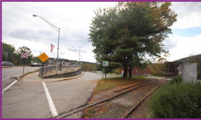
Justus Park's Main Vehicular Entrance on Western Edge of the Veterans' Memorial Bridge
