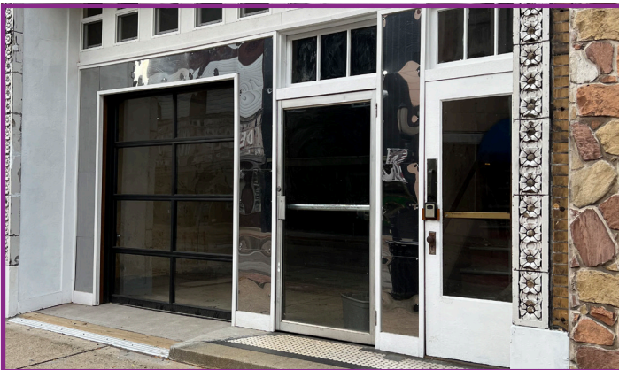
Historic Commercial Building Altered by Inappropriate Fenestration Pattern
