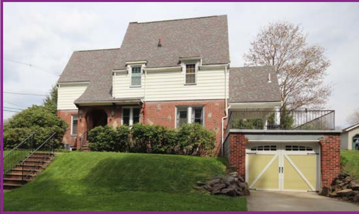
Stairs Built Into Slope
