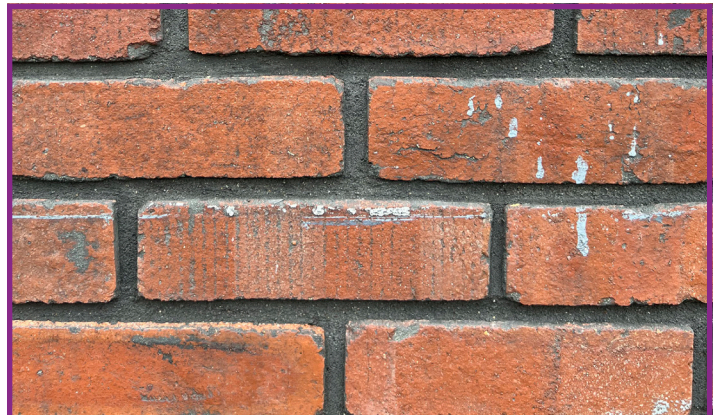
Masonry Before and After Repointing
