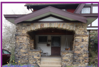
Stone Entry Porch
