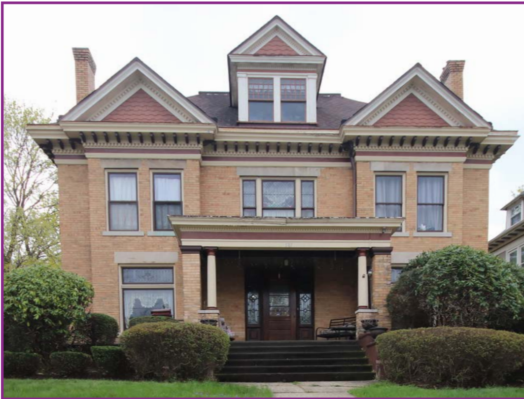
CLASSICAL REVIVAL South Side Historic District, Third Street
