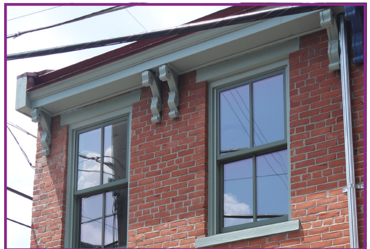
Before and After of Painted Wood Trim and Detailing
