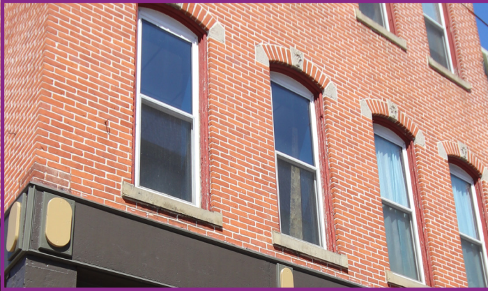
Well Maintained Masonry
