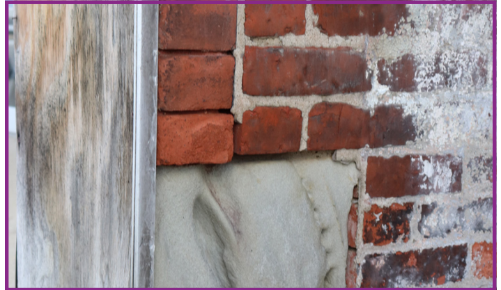
Inspect Brickwork, Mortar and Stonework
