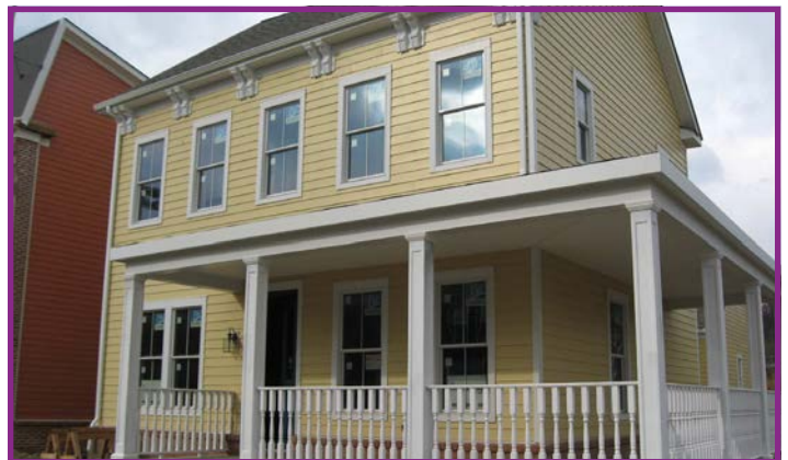
New House on a Corner has a Wrap-Around Porch to Address the Secondary Frontage, but is More Prominent on the Primary Frontage
