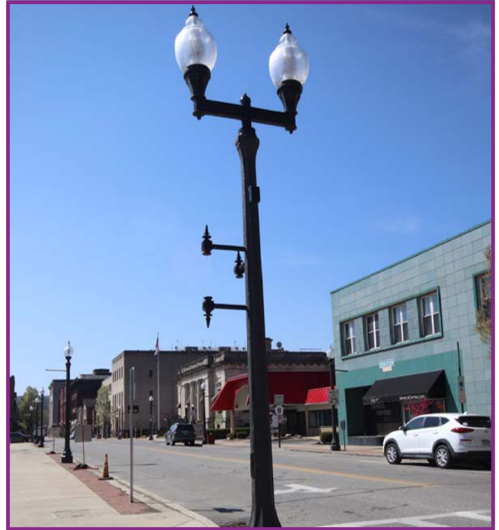
Existing Street Lights
