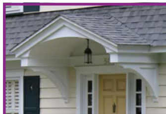
Hood Entry with Bracketed Pediment
