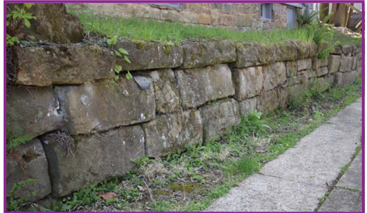
Boulder Retaining Wall
