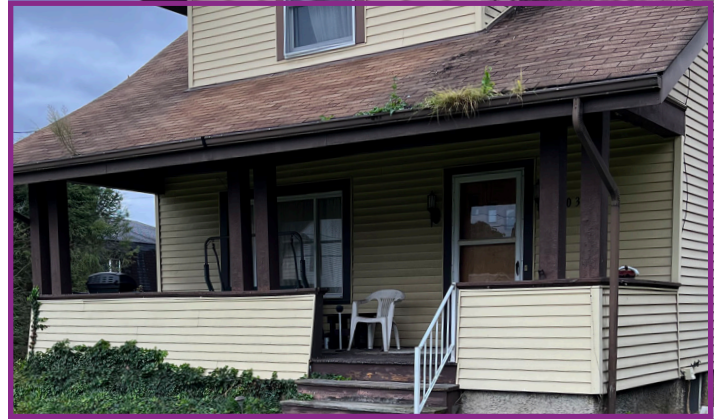
Clean Gutters and Inspect Roof Shingles
