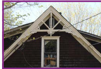
Trusses in Gable
